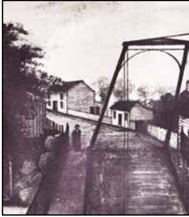
Early Pocahontas Bridge
