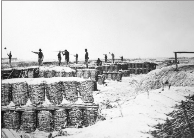
Gabions - cages filled with earth or rocks
