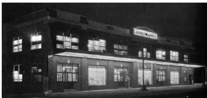
The Electric Building when it opened in 1926
