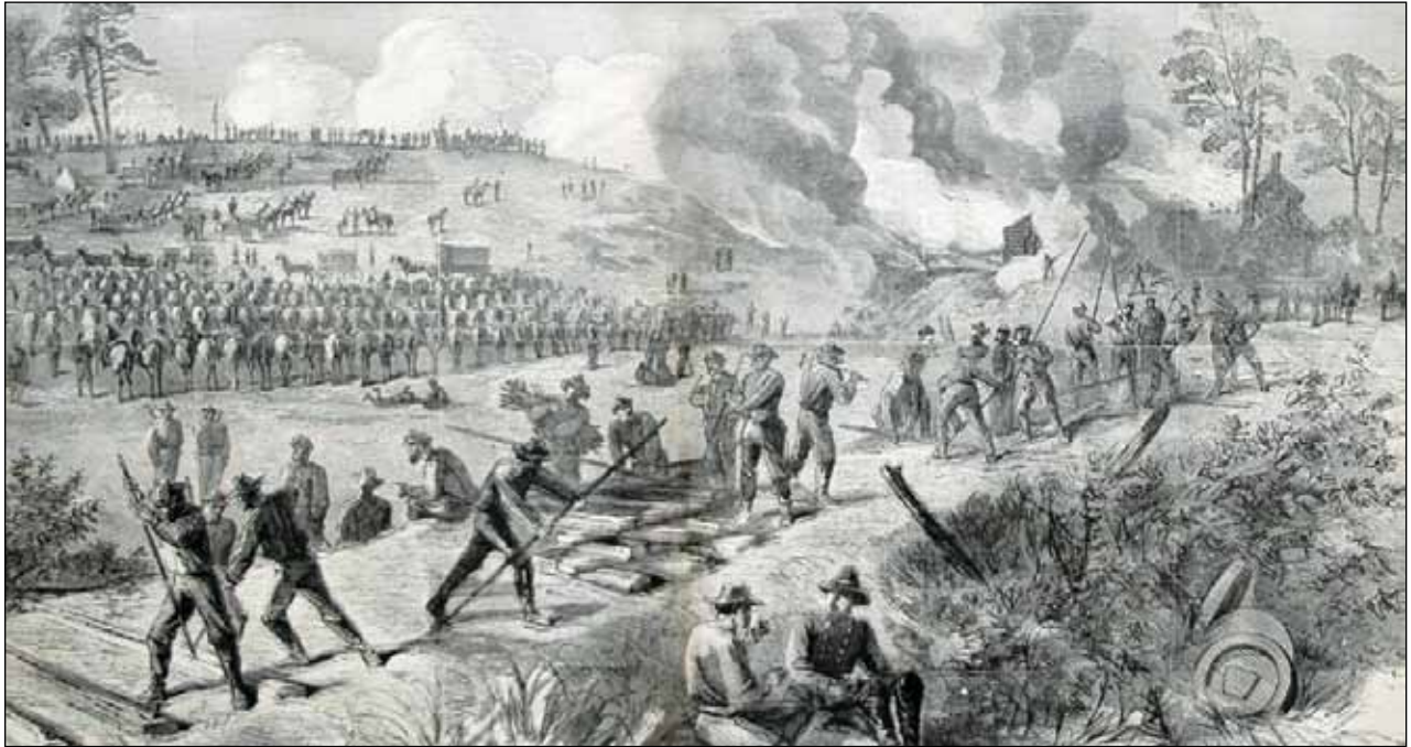
Tearing up the track
